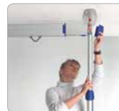
Fix end cap to lock rail in place.
